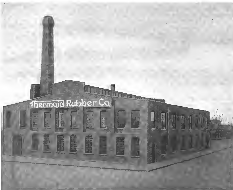
New Brick and Steel Building of the Thermoid Rubber Company at Trenton, N. J.
